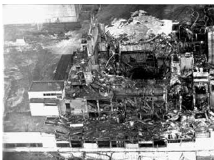
April 26, 1986 during the trial of one of the technological regimens, about 1:23 there was an explosion, which completely destroyed the reactor N4
