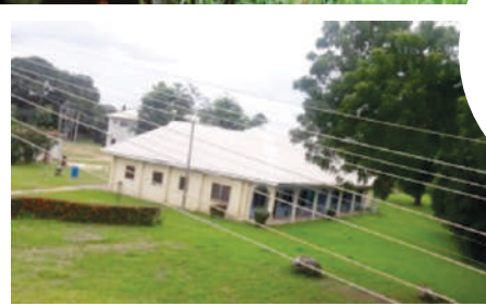
Mile Four Hospital, Abakaliki
